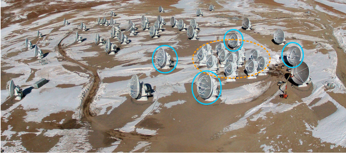
Figure 2.1: The ALMA 12-m Array in its compact configuration (left hand side of the image). The ACA with all 7-m antennas (dashed orange circles) and four single-dish 12-m antennas (blue circles) are distributed in the right hand side of the image. A few unoccupied stations can be seen, to which antennas of the 12-m Array can be moved by the transporter as the array is being reconfigured. At its most extended configuration, antennas in the 12-m Array will be about 16 km apart.
