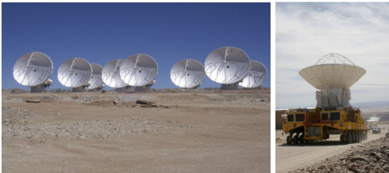
Figure A.3: The ALMA array with eight 12-m antennas (left), and an antenna being transported to the AOS (right).
