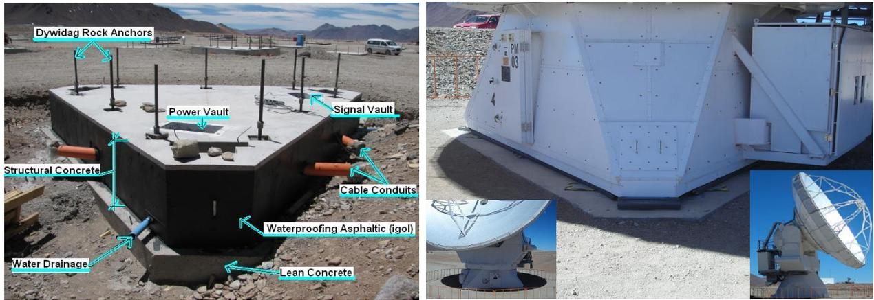
Figure 65. Structure of an antenna pad (actual pad at the OSF) (left) and detail of antenna anchored to a pad (right).
