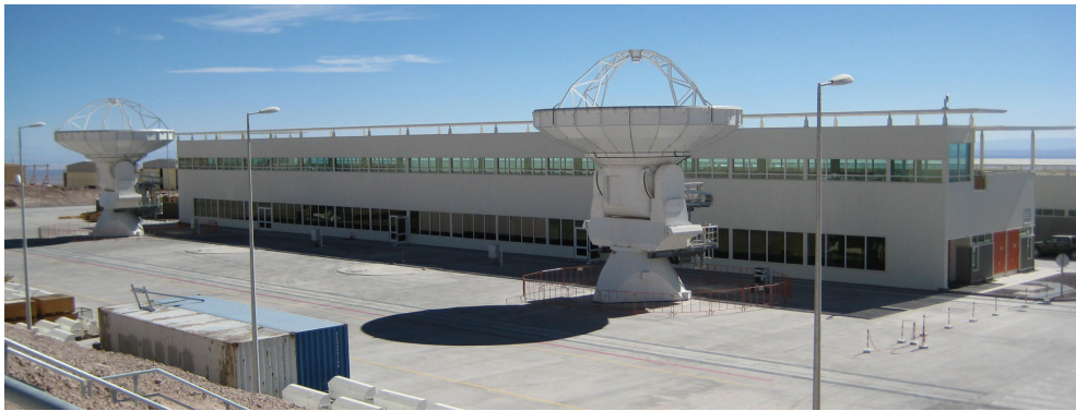
Figure 3: Operations Support Facility (OSF). Inside this building are offices, receiver labs, conference rooms, and the Array control room. In front are two antennas being commissioned. Photo courtesy J. Di Francesco.
