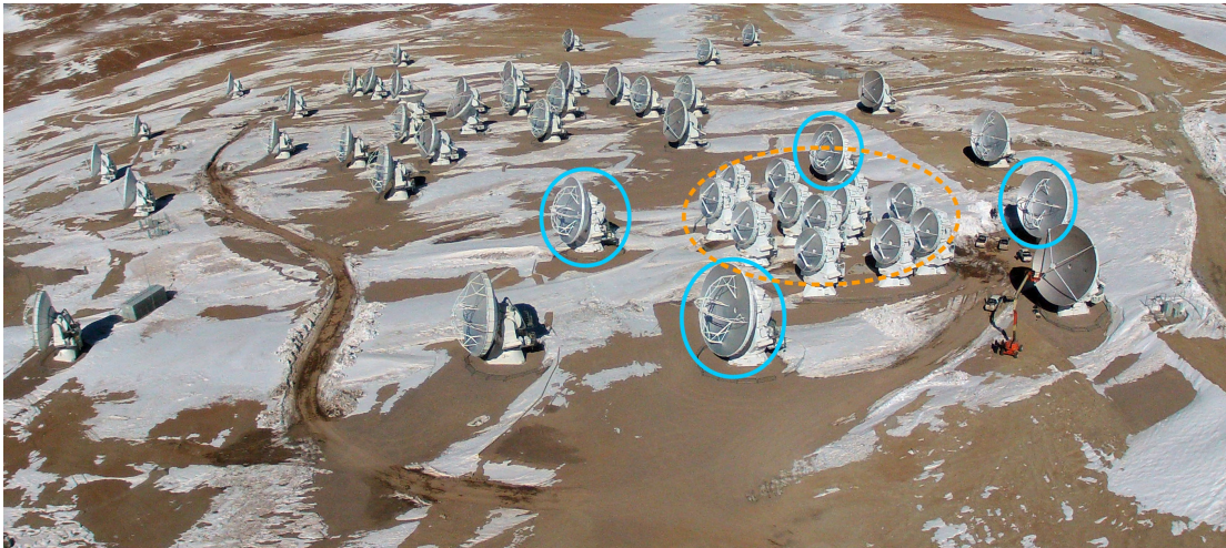
Figure 2.1: The ALMA 12-m Array in its compact configuration (left hand side of the image). The ACA 7-m Array with all 7-m antennas (dashed orange circles) and four single-dish 12-m antennas in the TP Array (blue circles) are distributed in the right hand side of the image. A few unoccupied stations can be seen, to which antennas of the 12-m Array can be moved by the transporter as the array is being reconfigured. At its most extended configuration, antennas in the 12-m Array will be about 16 km apart.
